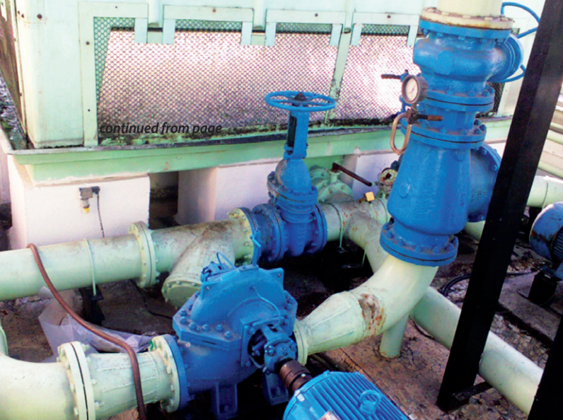
After energy audit at a site in Mumbai, 22 kW condenser water pumps (left) were replaced with 7.5 kW pumps (right)
