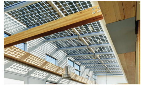
Figure 13: Building Integrated Photovoltaic (BIPV Solar Glass skylight) at Centre for Interactive Research on Sustainability - designed to be the most sustainable building in North America.
