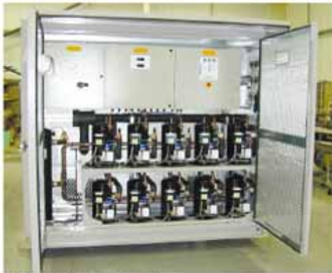
A typical Scroll rack.
