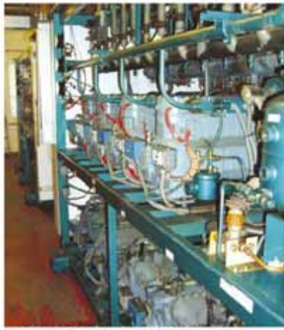
A typical Semi-Hermetic rack.
