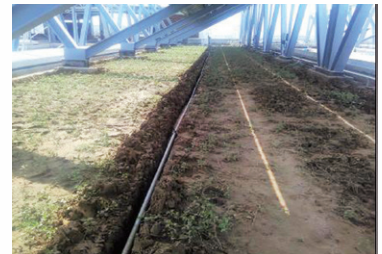
Roof top vegetation
