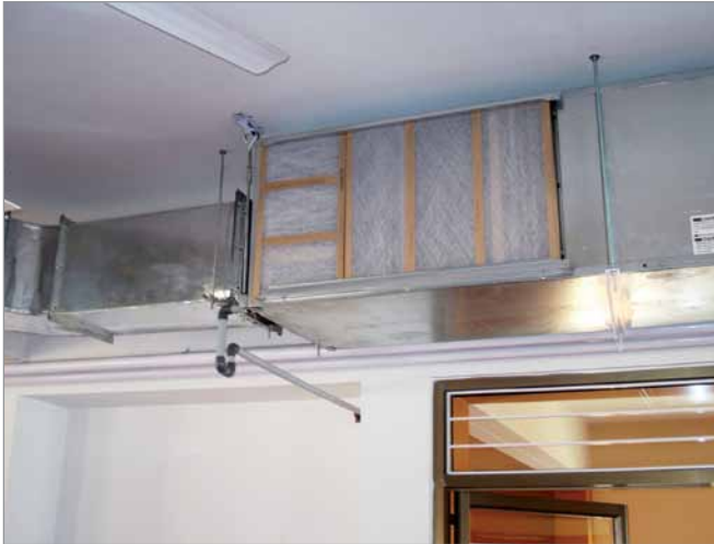
Figure 3: ClimateMaster GR060 vertical unit suspended from ceiling
