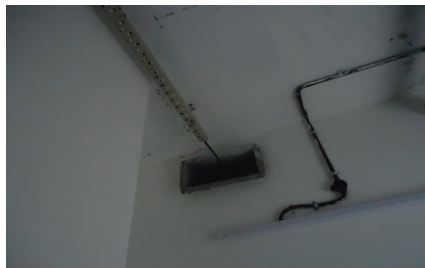
Photo 12: Cable passing through duct
