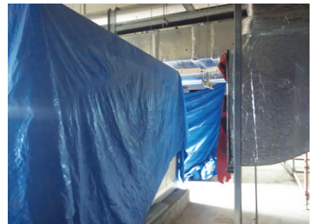
Photo 4: Equipment covered during construction
