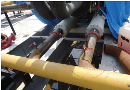
Photo 7: Shoe piece provided to reduce friction loss
