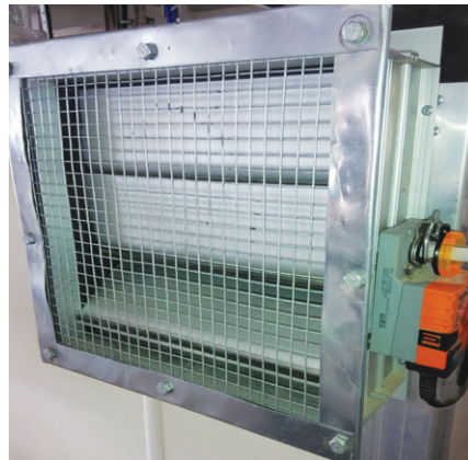
Photo 1: Anti-bird net for safety
