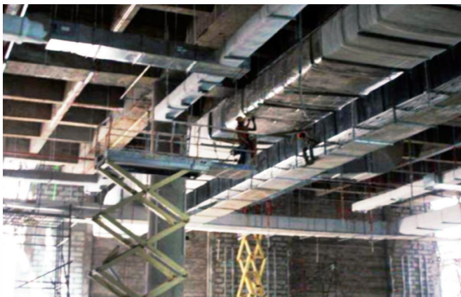
Photo 9: Ducting and insulation work in progress in immigration area with battery operated scissor lifts
