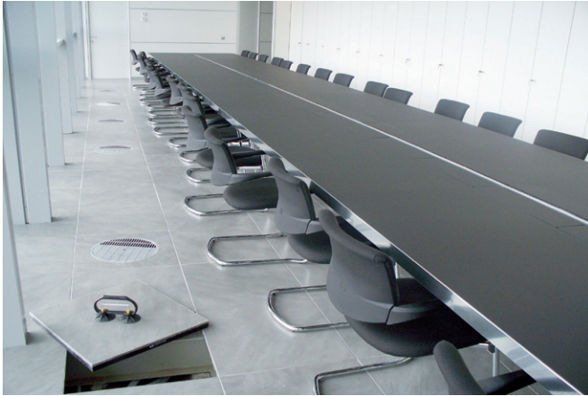
Figure 2: Air terminal units replace floor panels
