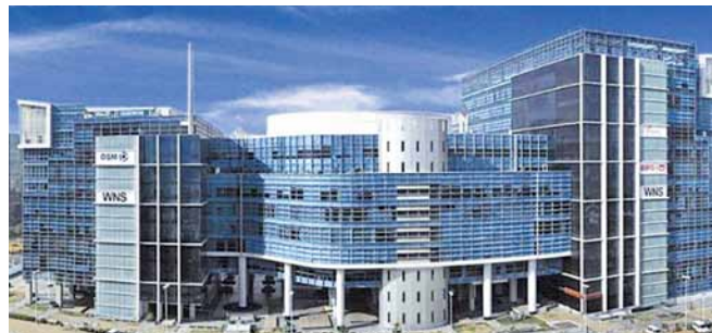
Photo 4: DLF Infinity Tower - 10MWe BCHP plant
