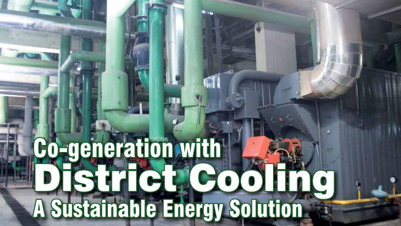
Photo 1: A battery of exhaust fired VAMs installed in a DLF building in Gurgaon
