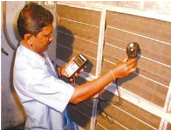
Air quantity recorded with filter before cleaning the coil.
