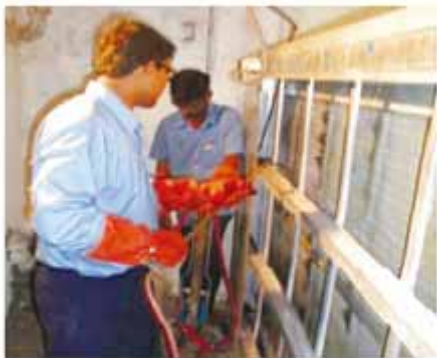
Spraying the coil with cleaning chemical.
