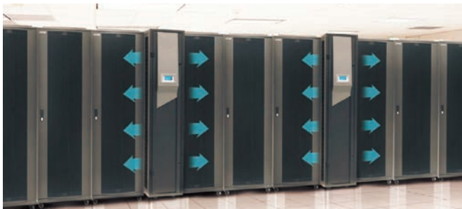
Figure 4: In-row cooling
