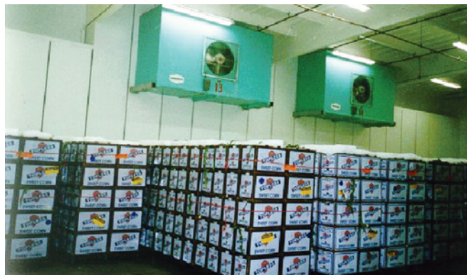
Photo 3: After precooling, grapes are stored in a cold storage maintained at 0^{\circ}\text{C} & 90% RH ready for loading in a refrigerated container for the journey by road to Mumbai port.
