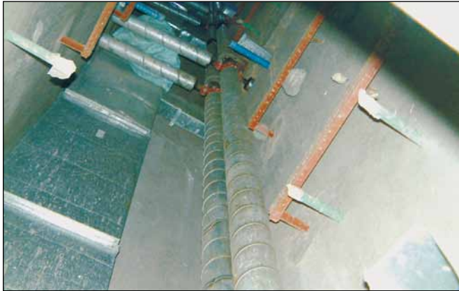
Photo 10 : Shaft insulation with pre insulated pipes.
