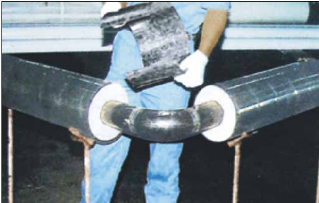
Photo 7 : Pre-insulated pipe lengths with field insulated elbow.
