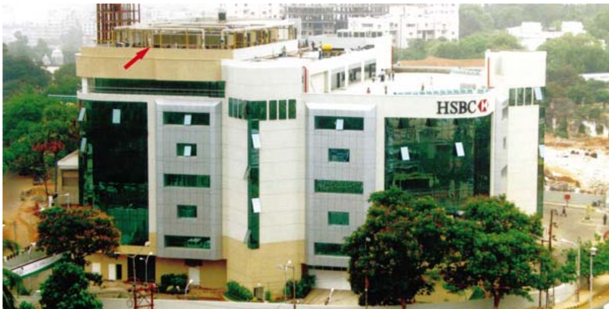
Photo 1: External view of a large data processing centre in Visakapatnam. Notice all the VRF units and chillers mounted on the terrace.
