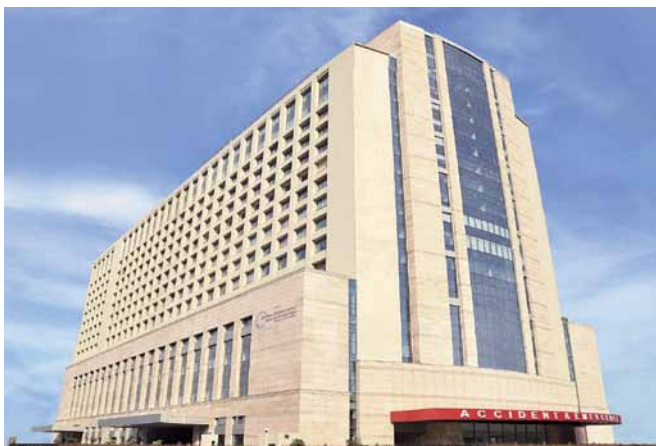
Kokilaben Dhirubhai Ambani, Mumbai, completed in 2009 with 700 beds & 21 OTs. Installed chiller capacity 3000 TR.
