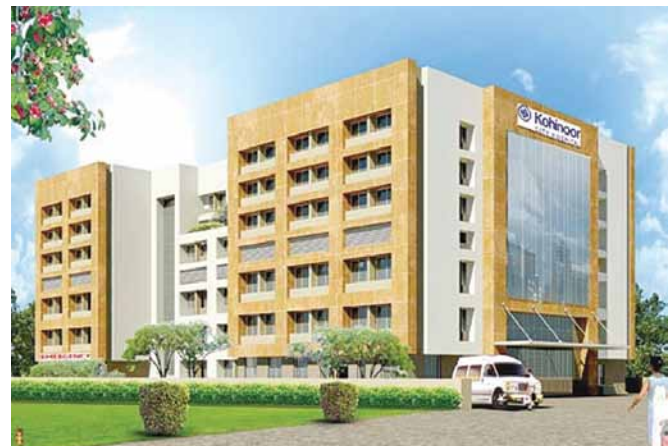
Kohinoor, Mumbai, completion in 2010 with 150 beds & 5 OTs. Installed chiller capacity 600 TR.
