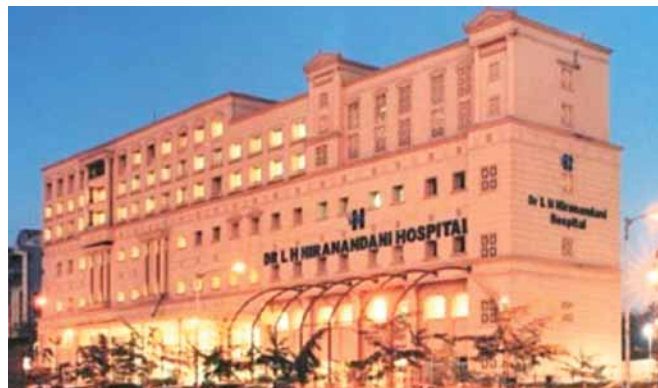
Hiranandani, Mumbai, completed in 2009 with 100 beds & 4 OTs. Installed chiller capacity 400 TR.
