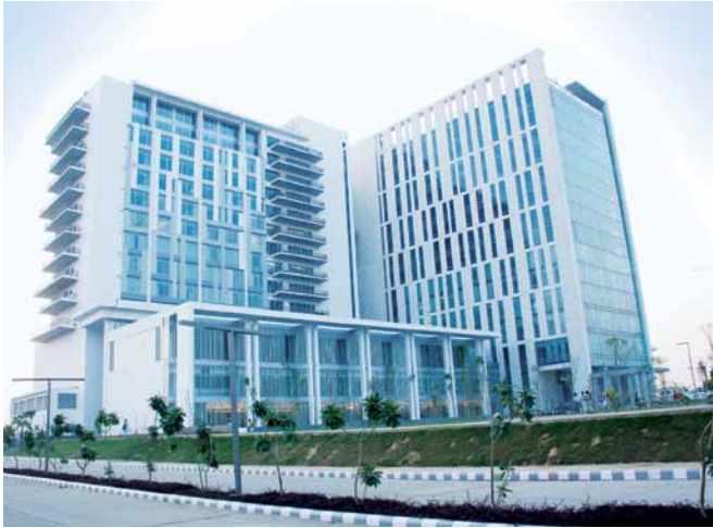
Medanta – The Medicity, Gurgaon, when fully completed in 2010, will have 1600 beds - 1250 normal, 350 critical care & 45 OTs. Installed chiller capacity 4800 TR. Photo & other details courtesy of Manish Bhatia
