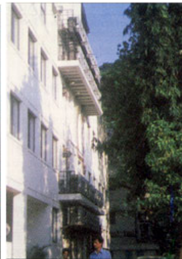
Photo 3: Air cooled condensing units mounted on a special RCC platform
