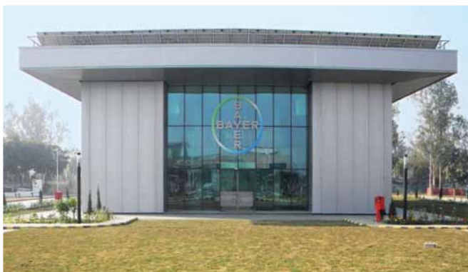
Photo 1: A front view of the Bayer building
