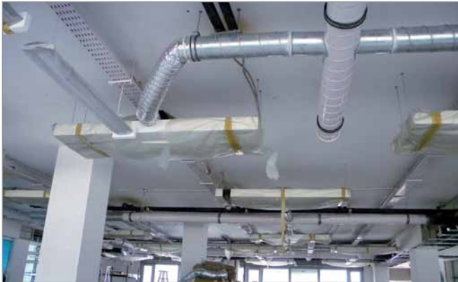
Photo 4: Installation of chilled beam
