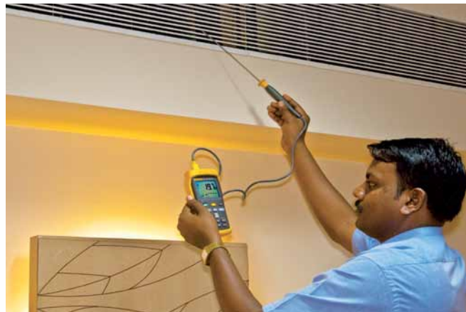
Grille air temperature measurement using air probe and thermocouple thermometer
