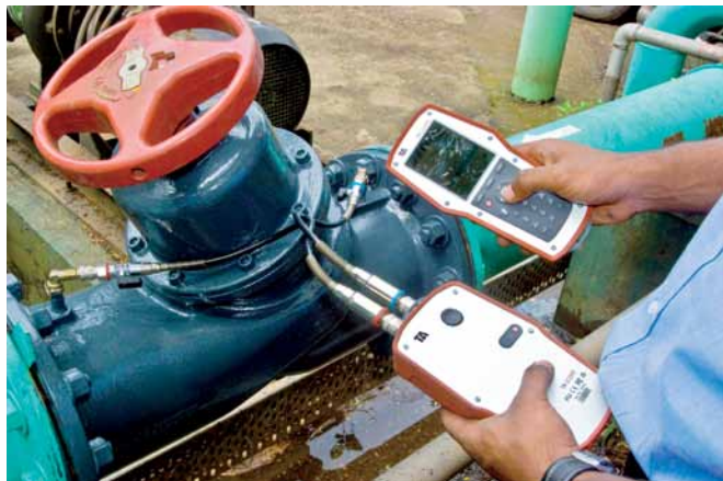
Water flow measurement using a differential manometer
