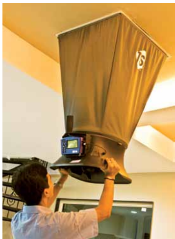
Cfm measurement at diffusers using an air volume hood
