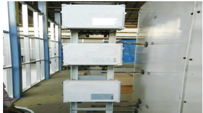
Photo 4: AHU control kit for three ODUs, three evaporator coils and three AHUs
