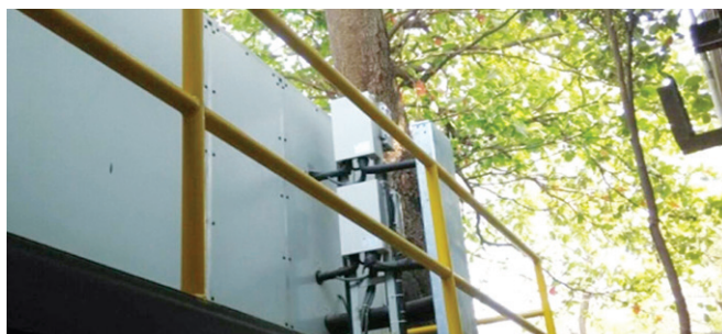
Photo 3: AHU control kit for two ODUs
