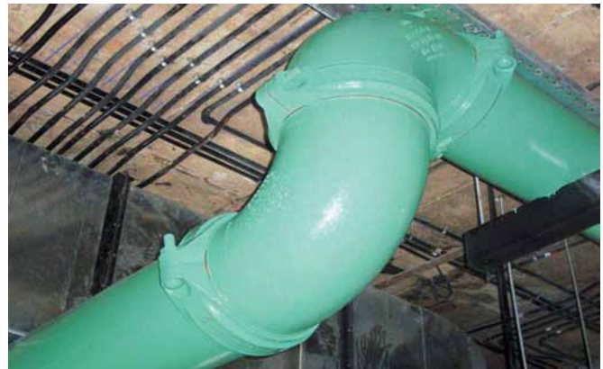
Photo 3: Grooved pipe joint installation in The Park Hotel Hyderabad
