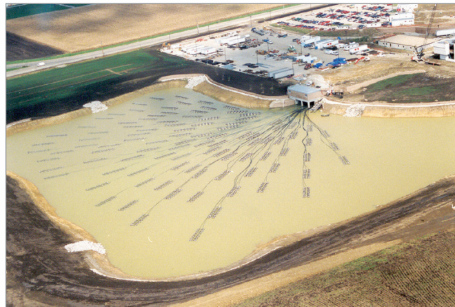
Photo 1: Installation of geothermal pond heat exchanger for a new hospital.
