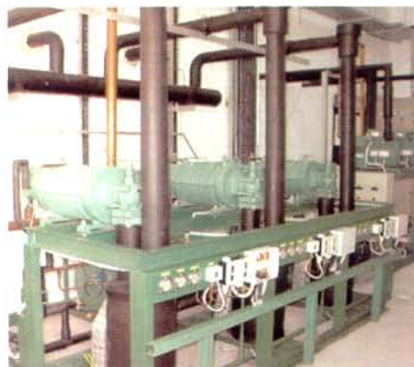
Figure 6: A rack with screw compressors
