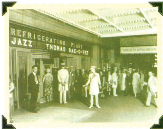
Photograph 2: Rivoli Theater in New York, 1925. This was an early centrifugal chiller installation, cooled by “refrigeration plant” as evidenced on the marquee. Photo credit: Carrier Corporation.
