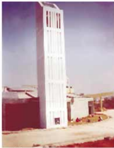
Figure 1: Tower for pre-cooling fresh air.
