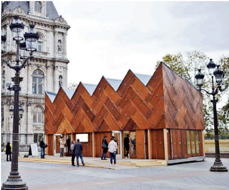
The Circular Pavilion, an experimental construction built with reusable materials on the forecourt of the City Hall in Paris for COP-21.
