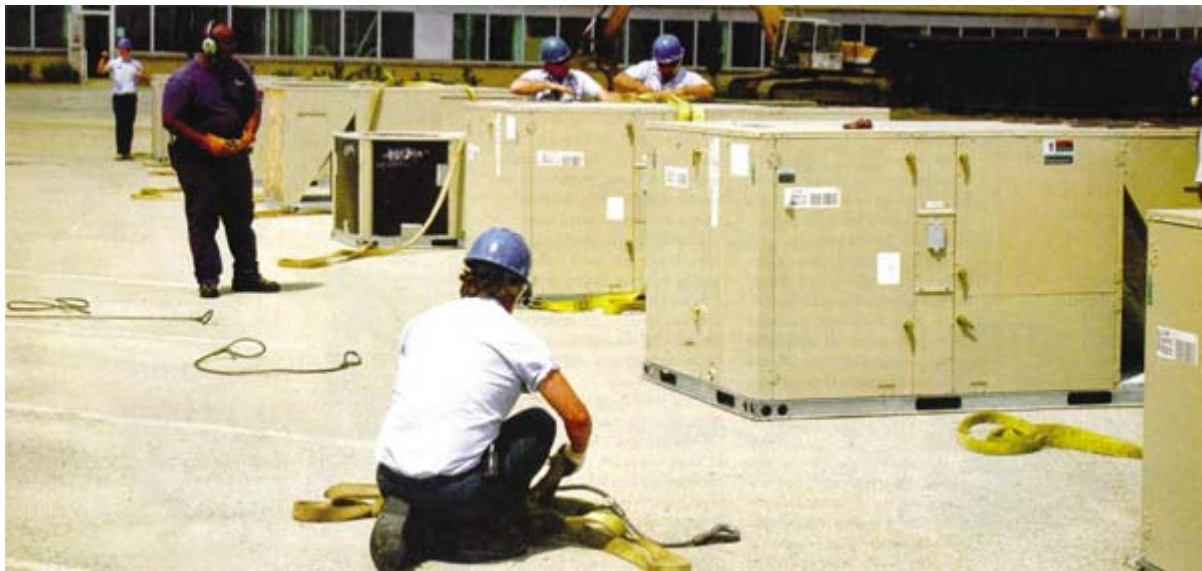
Photo 1 : Rooftop units under installation in the USA.
