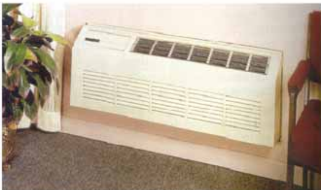
A typical PTAC unit.
