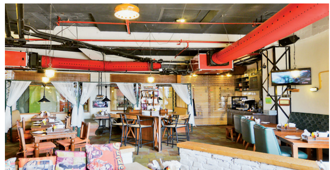
Figure 4: Conventional fabric duct without in-duct tensioning in a restaurant
