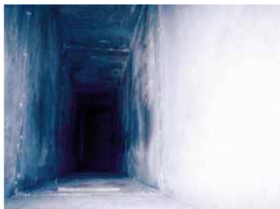
The same duct after cleaning.
