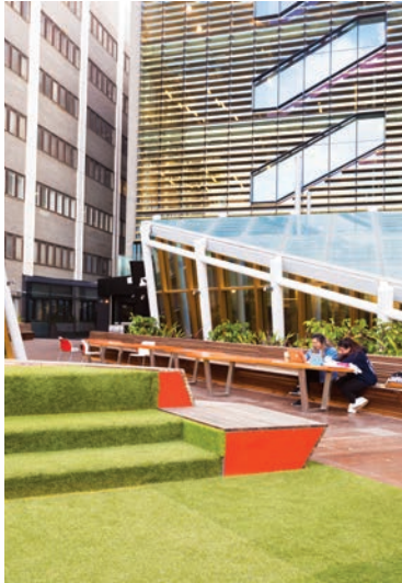
Building 10, Level 7 roof terrace and theatre stack
