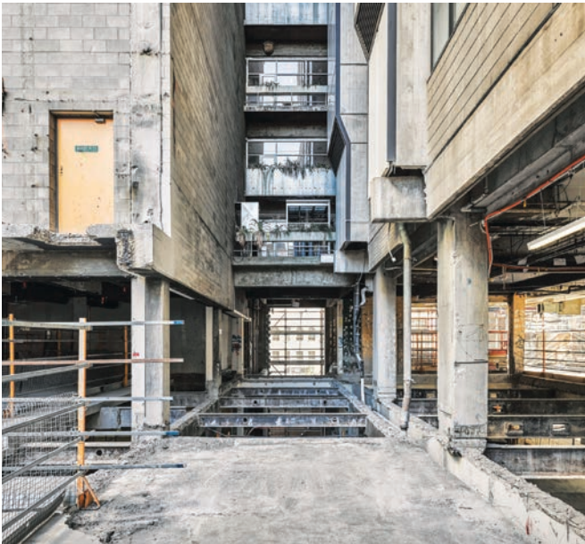
Building 14, Level 4 during construction
