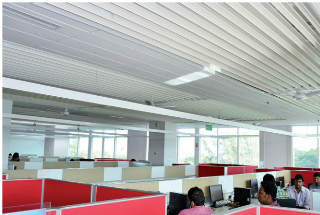
Figure 1: Radiflux panels installed in Infosys building in Bangalore
