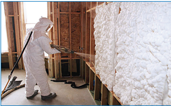
Figure 3-20: Spraying of polyurethane, and filling cracks in cold room floors
