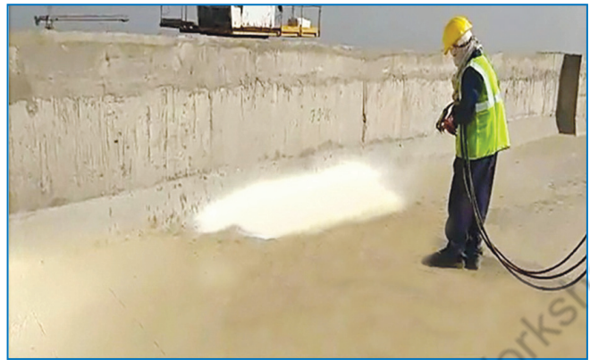
Figure 3-20: Spraying of polyurethane, and filling cracks in cold room floors
