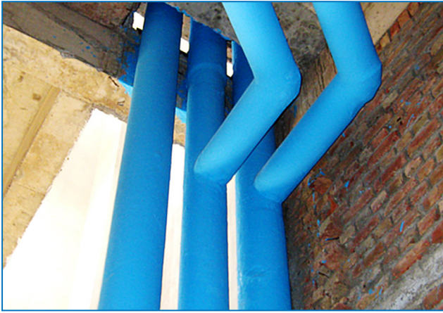
Figure 6-30: Vapour barrier mastic coating paint applied over pipe insulation
