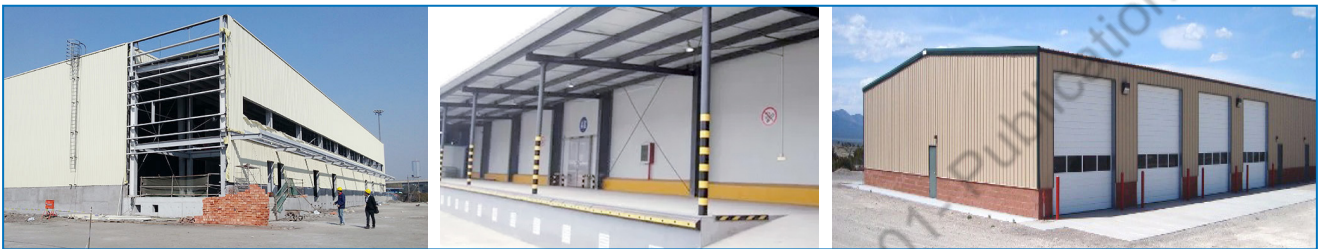
Figure 3-29: Cold storages with continuous panels and steel structure under construction
