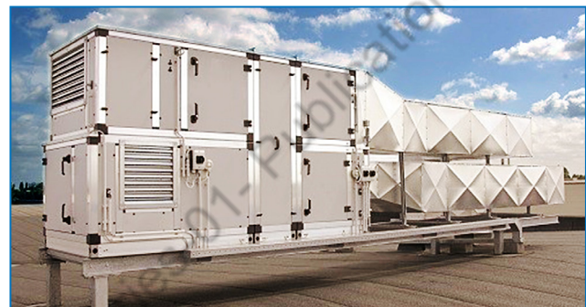
Figure 7-2: AHU installed outdoors
