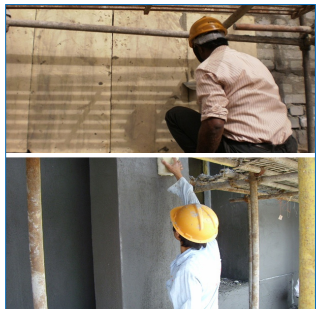
Figure 5-14: Revamping of walls
