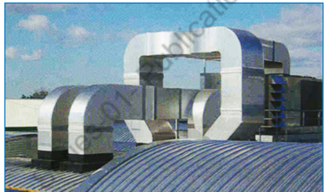
Figure 7-4: Duct insulation
