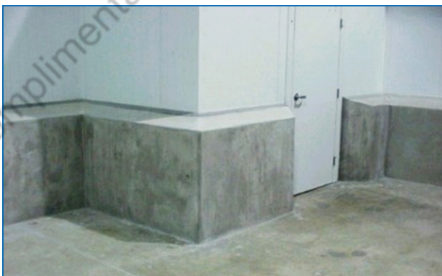
Figure 5-29: Curb wall of concrete to protect insulation panels
