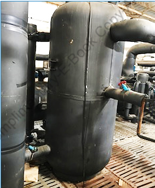
Figure 6-21: Inter-stage cooler in two stage system
