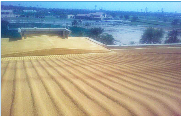
Figure 3-21: Use of spray foam on roofs
