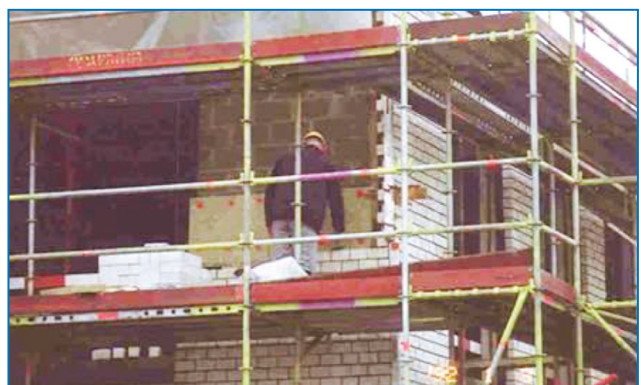
Figure 7-6: Cavity wall insulation
