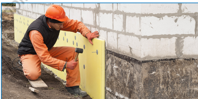
Figure 5-7: Application of EPS to wall
