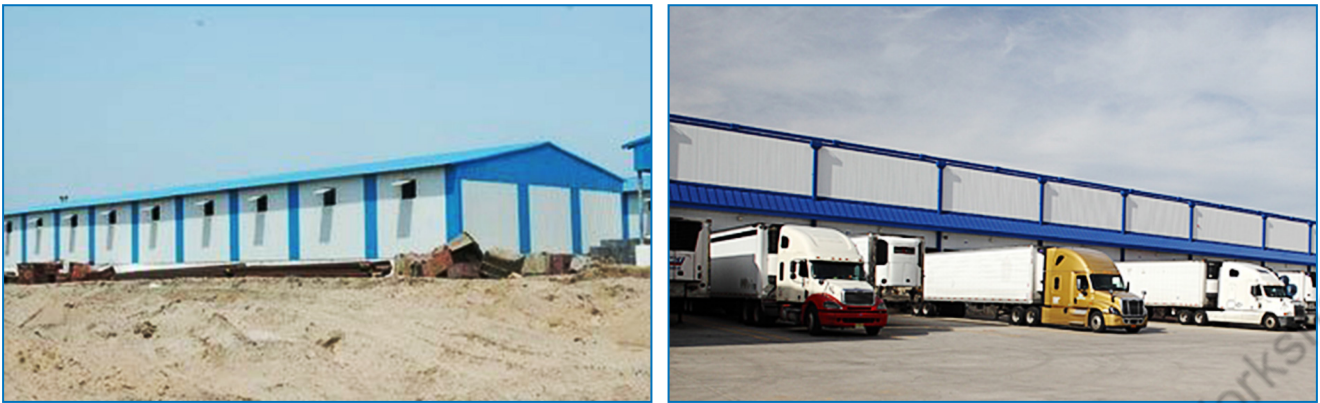
Figure 3-28: Cold storages with continuous panels and steel structure
