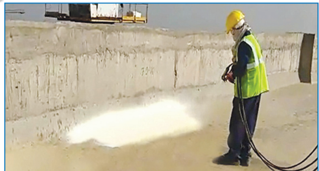
Figure 7-5: Insulation sprayed on roof
