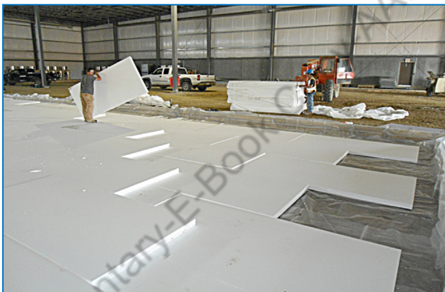
Figure 5-6: Application of EPS to floor
