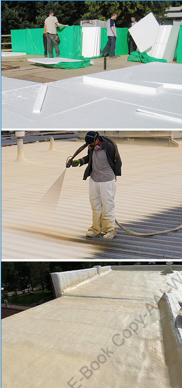
Figure 5-15: Revamping of roof
