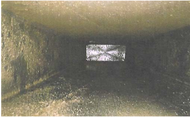
Figure 5: Duct condition before and after cleaning
