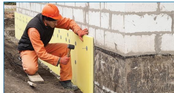
Figure 5-8: Application of PUF to wall
