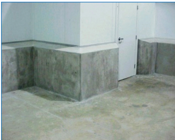
Figure 5-29: Curb wall of concrete to protect insulation panels
