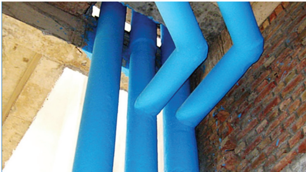
Figure 6-44: Vapour barrier mastic coating paint applied over pipe insulation
