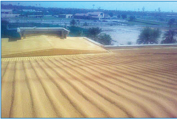
Figure 3-20: Use of spray foam on metal roofs
