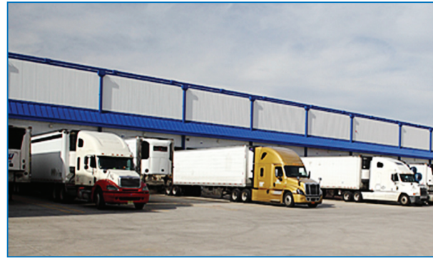
Figure 3-28: Cold storages with continuous panels and steel structure
