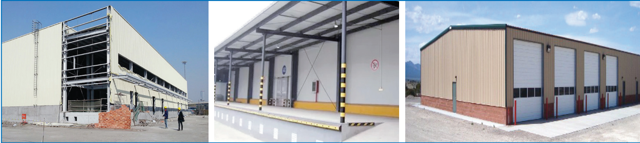
Figure 3-29: Cold storages with continuous panels and steel structure
