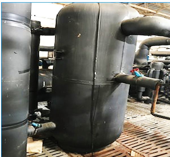
Figure 6-25: Inter-stage cooler in two stage system
