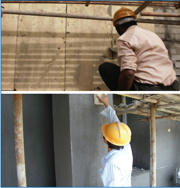
Figure 5-14: Revamping of walls
