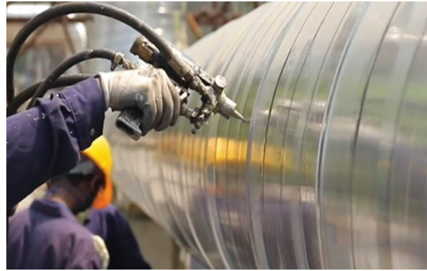
Figure 6-38: Injecting PU Chemicals
