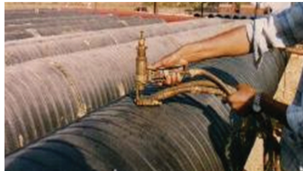
Figure 6-39: HDPE Cladding & Injection
