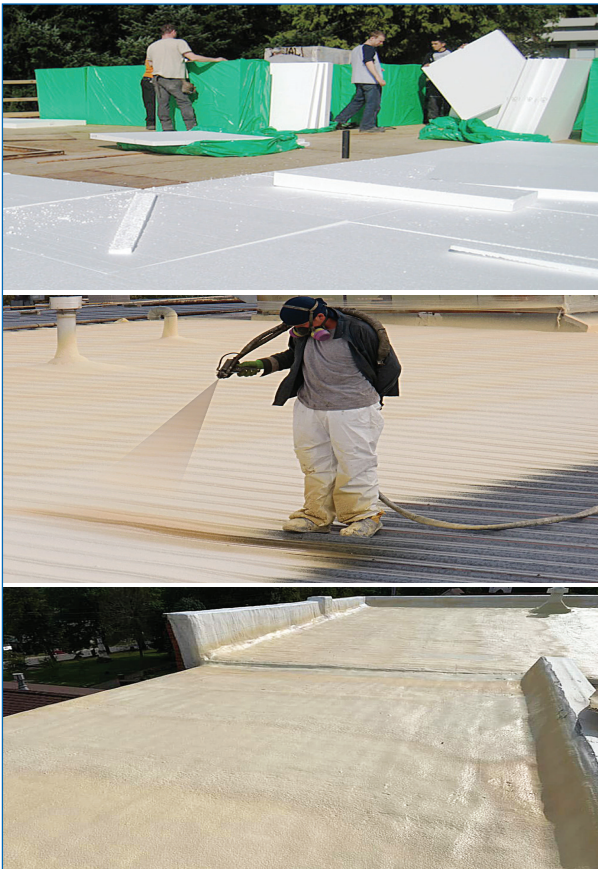
Figure 5-15: Revamping of roof with Sprayed Polyurethane Foam Insulation
