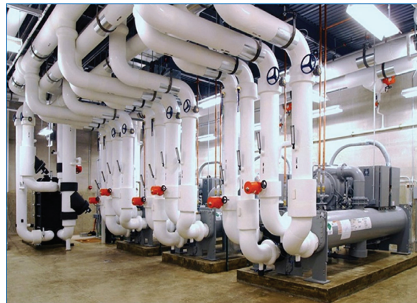
Figure 6-45: Application over pipe insulation
