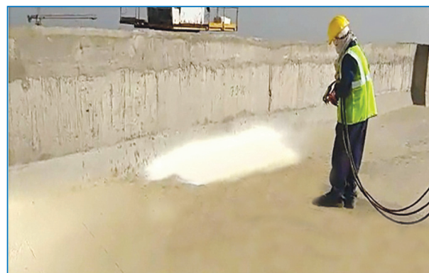
Figure 3-19: Spraying of polyurethane, and filling cracks in parapet Walls & Roof of Buildings & Cold Stores
