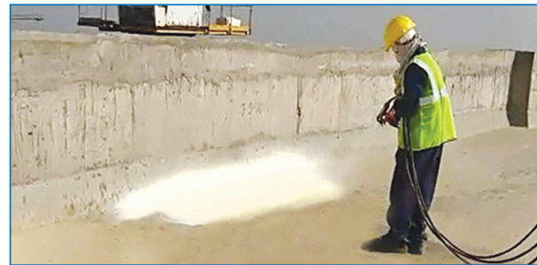
Figure 7-5: Insulation sprayed on roof
