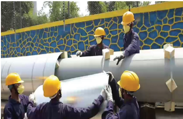
Figure 6-37: Fixing Spacers & Sheet
