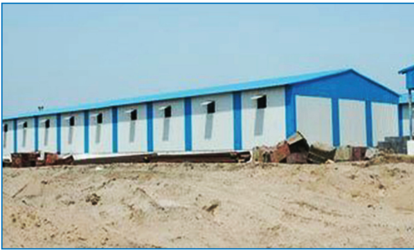
Figure 3-28: Cold storages with continuous panels and steel structure
