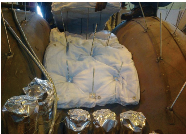
Figure 6-40: Turbine Insulation with Pads
