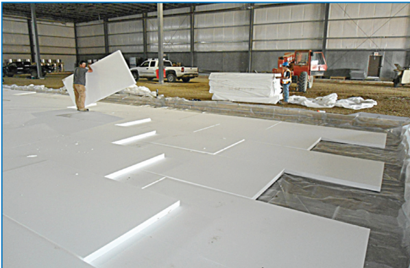
Figure 5-6: Application of EPS to floor
