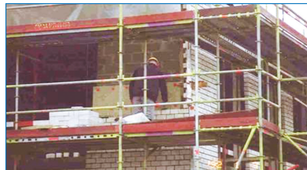
Figure 7-6: Cavity wall insulation
