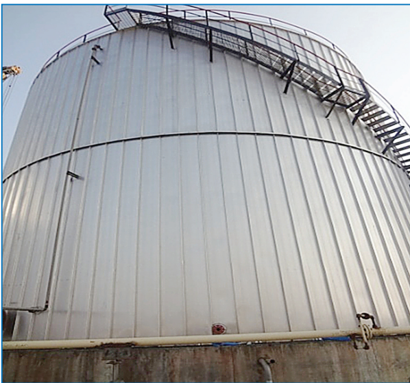
Figure 6-32: Pre-insulated tank
