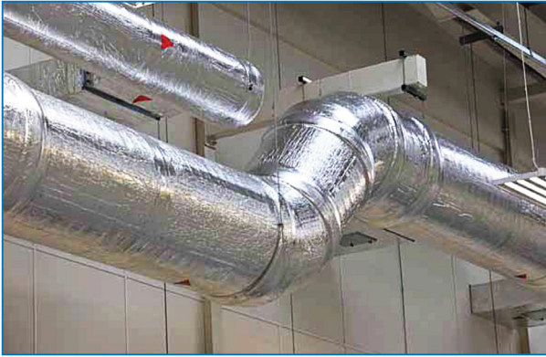
Figure 6-31: Insulation protected by aluminium foil lamination vapour barrier
