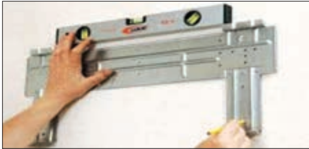
Figure 3.8: Template for marking drilled holes for fixing indoor unit
