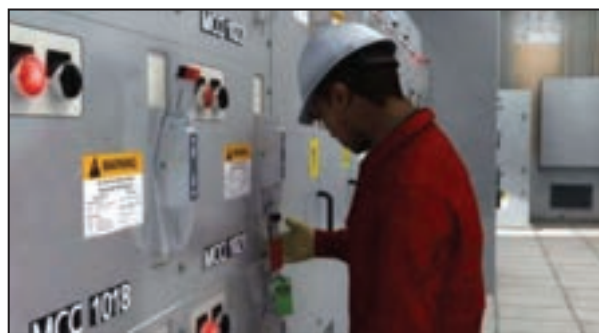
Figure 21.5: Working on electrical panel
