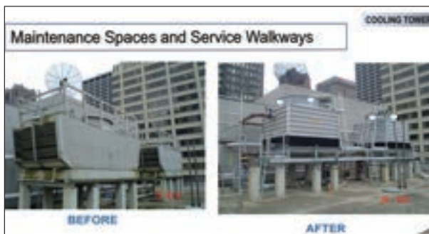
Figure 6.9: Maintenance walkways make the tower serviceable
