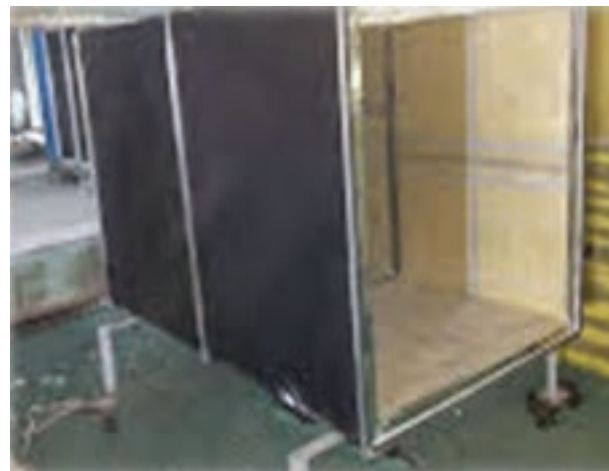
Figure 13.9: Duct acoustic insulation with glass wool
