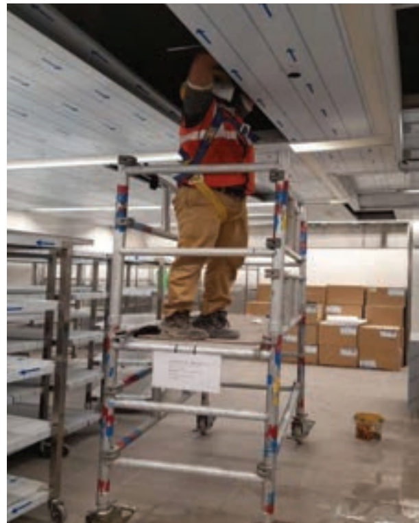
Figure 21.2: Working at height with scaffolding
