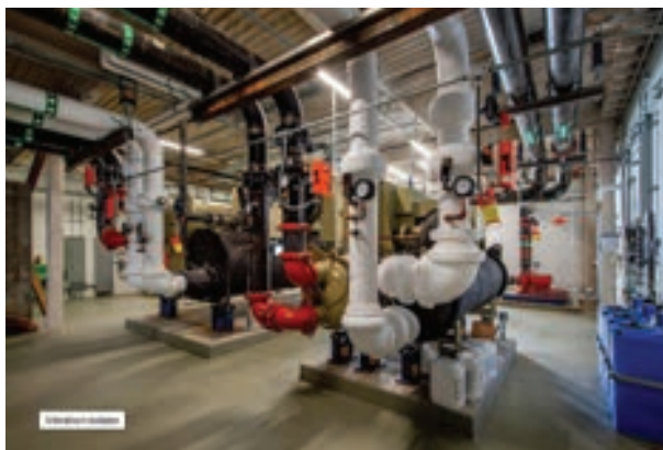
Figure 5.1: Water cooled chiller with vibration isolator
