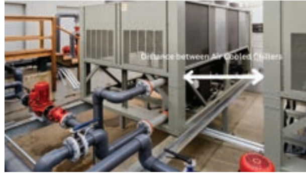
Figure 5.2: Air cooled chiller – multiple units with spacing
