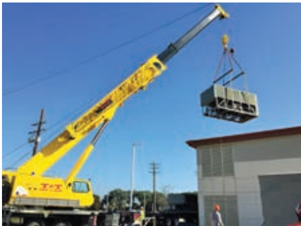
Figure 2.1: Typical lifting of chillers with crane
