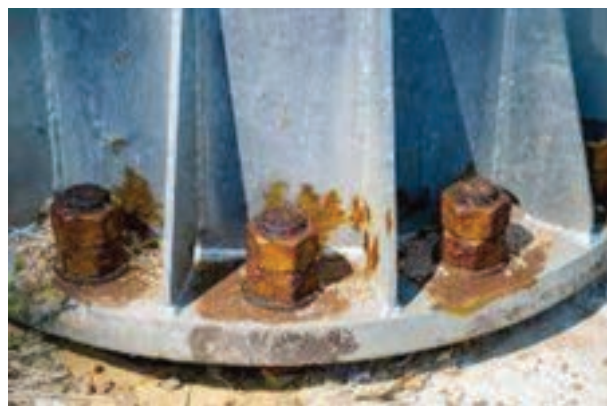
Figure 20.1: Galvanic corrosion
