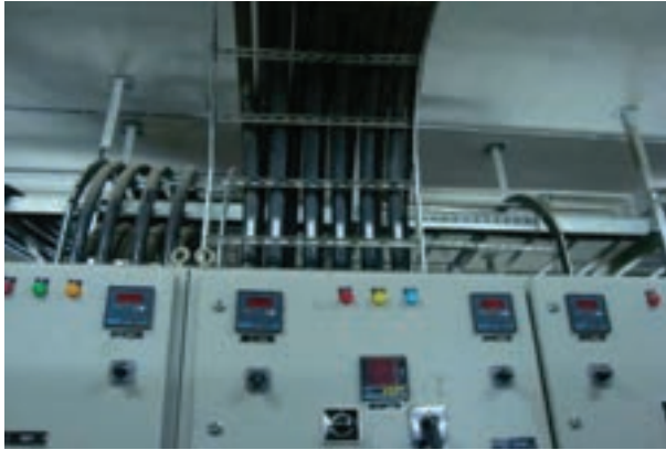
Figure 17.3: Termination of cables
