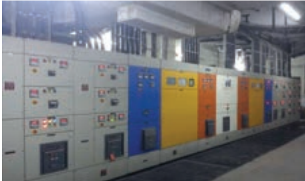
Figure 17.1: Electrical panel installation
