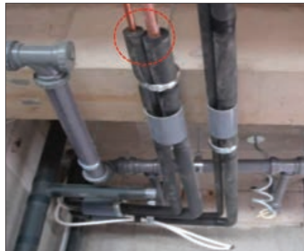
Figure 4.21: Insulation of refrigerant piping
